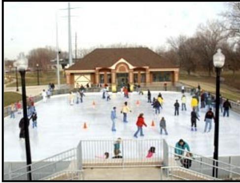
**Tapawingo Skating Rink.** The rink and pavilion were constructed on an engineered fill to raise the site to level with Tapawingo Drive. The project included the construction of reinforced slab on grade with cooling tubes and accessories, perimeter rail, dasher boards, site utilities, and a monumental stair which links the rink to the Margerum Fountain located at the entrance to Tapawingo Park.
