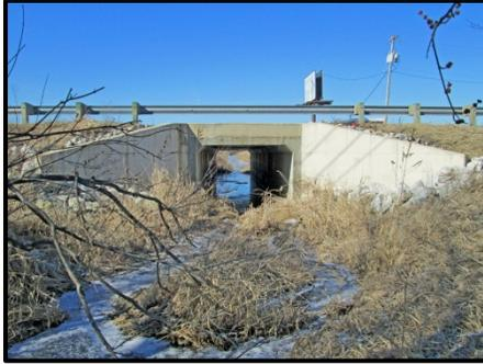
**US 41 over Feddeler Ditch, Lake County, Des. No. 0014130:** This box culvert replacement under the four lane US 41 highway involved phased construction with maintenance of two lanes per phase.
