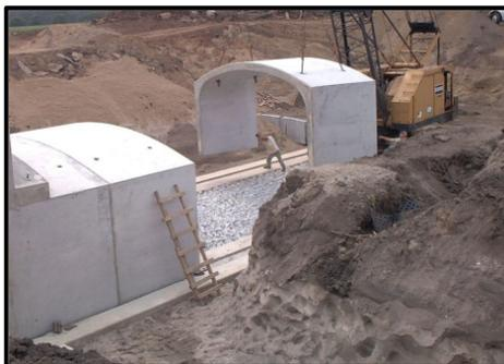
**Tippecanoe County 3-Sided Culvert:** The 28 ft. structure was designed to replace an existing undersized culvert. The structure was sized and constructed as part of a new open legal drain in an urbanizing area. The barrel length and headwalls were designed to allow for the future construction of a four lane urban street with sidewalks.
