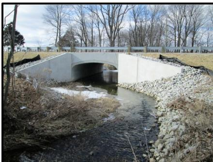
**SR 32 over Indian Camp Creek, Madison County, Des. No. 0101420:** This 2011 three-sided structure on a super elevated curve adjacent to an intersection and a cemetery included 1000 ft. of approach roadway, right-of-way, phased traffic maintenance using a temporary signal, and a new storm drain. HSK also provided 401/404 and Rule 5 permitting.
