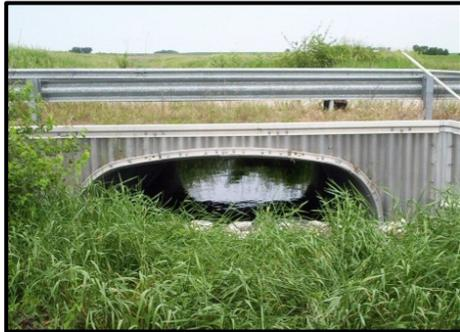
**Tippecanoe County Culvert JAC403:** The 14 ft. X 6 ft. aluminum box culvert carries a low volume (22 VPD) 18 feet wide gravel road over the Little Wea Conservancy and the Leader Newton tile. Given the low traffic volumes and isolated location it was determined that the aluminum box culvert would provide a low maintenance, long lived, long spanned alternative to multiple pipe culverts. The culvert was designed with a 35 ft. barrel length allowing for potential future roadway widening.
