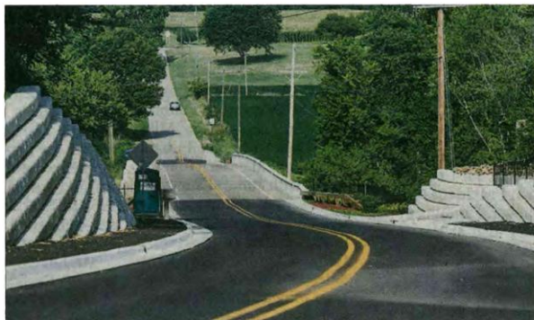
Pretty Prairie Road crosses Hog Point Bridge.
